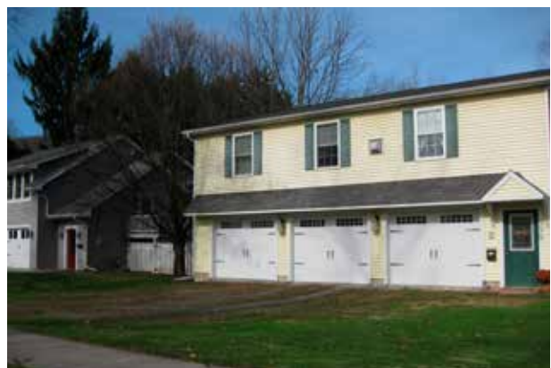
Example of an elevated home in the Tioga Community.
