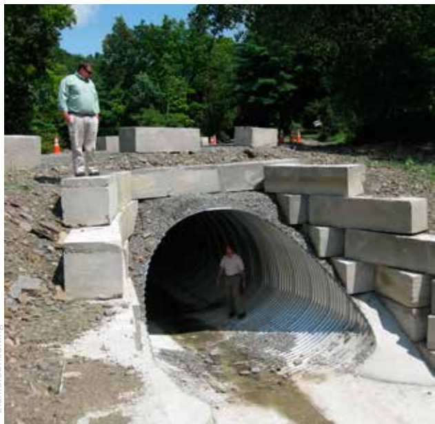
Many culverts were damaged and had to be replaced as a result of Tropical Storm Lee.
