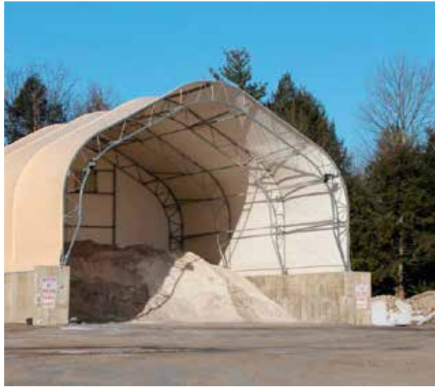
Typical salt storage facility and cover.
