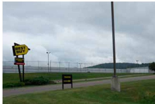
Sanitary sewer service is currently limited to the Best Buy Distribution Center and Army Reserve Center on Stanton Hill Road.
