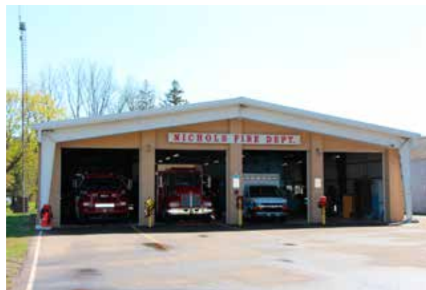
Existing Nichols Joint Fire Station.
