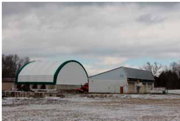
The Nichols Highway Garage suffered extensive damage during Tropical Storm Lee.
