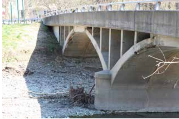
Example of a double culvert in Nichols.
