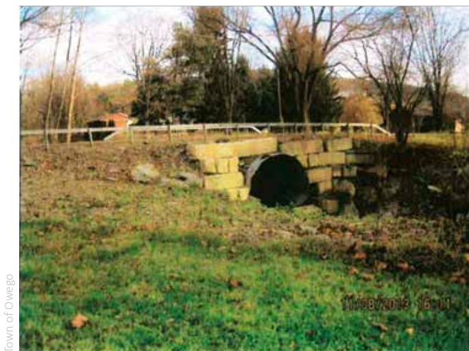
South elevation downstream of culvert.
