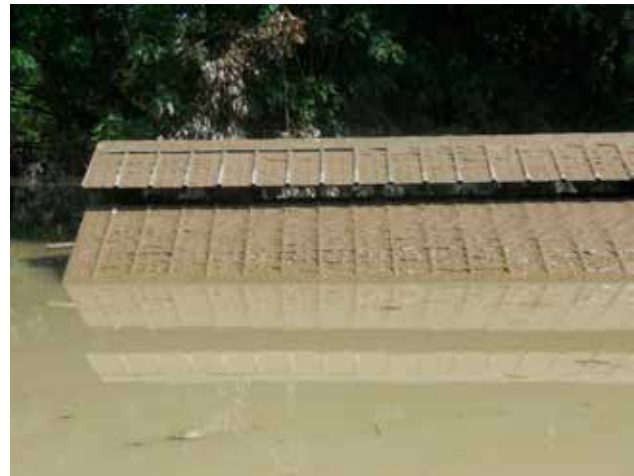
The flood covered 90% of Kirby Park in mud and silt.
