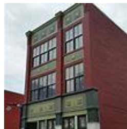
18 Lake Street, Owego (4 apts)
