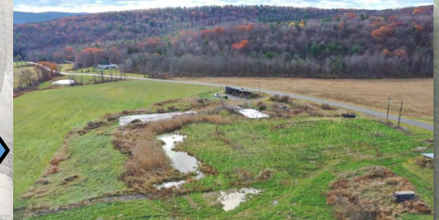
Barn Foundation Removed & Old Storage Pit was emptied and closed to turn it into a wetland complex - photo taken in November 2025
