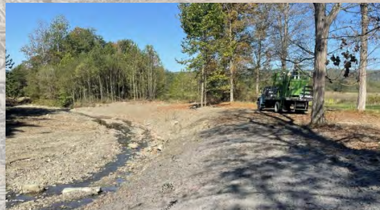
SWCD assisted the Town Water Department in permitting and technical oversight to re-build the stream bank and re-establish the proper stream dimensions. Large root balls and live willow stakes were installed to promote stability. Then SWCD hydroseeded the site.
