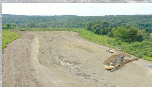
Construction of a flood control basin (during installation of the primary outlet pipe)—photo taken in August 2025
