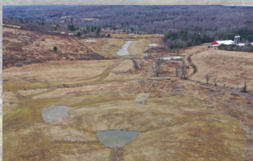
Completed basins along with wetland pools constructed by the USC - photo taken in March 2026 (looking from north)
