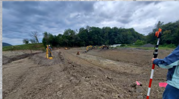
Construction & Stakeout of Waste Storage Facility in Truxton (Cortland County) - photo taken in September 2025
