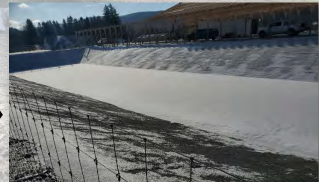
Completed Waste Storage Facility in Truxton (Cortland County) - photo taken in December 2025
